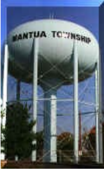
1 Million Gallon Storage Tank Main Street / Barnsboro
