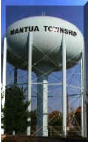
1 Million Gallon Storage Tank Main Street / Barnsboro
