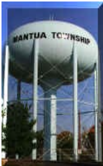
1 Million Gallon Storage Tank Main Street / Barnsboro
